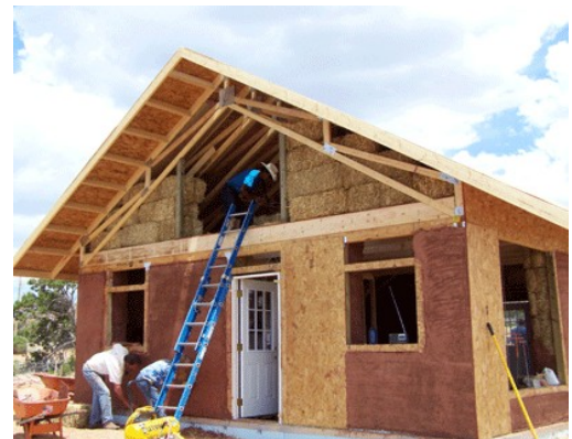
Straw-bale home we built in Window Rock, AZ.
