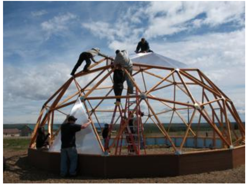
New Stuyahok Geodesic dome greenhouse
