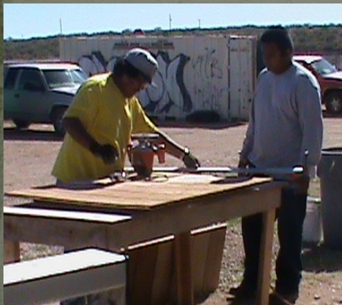
Vernon Hudson, Sr., carpentry With Ferris Irving, Sr., Site Supervisor
