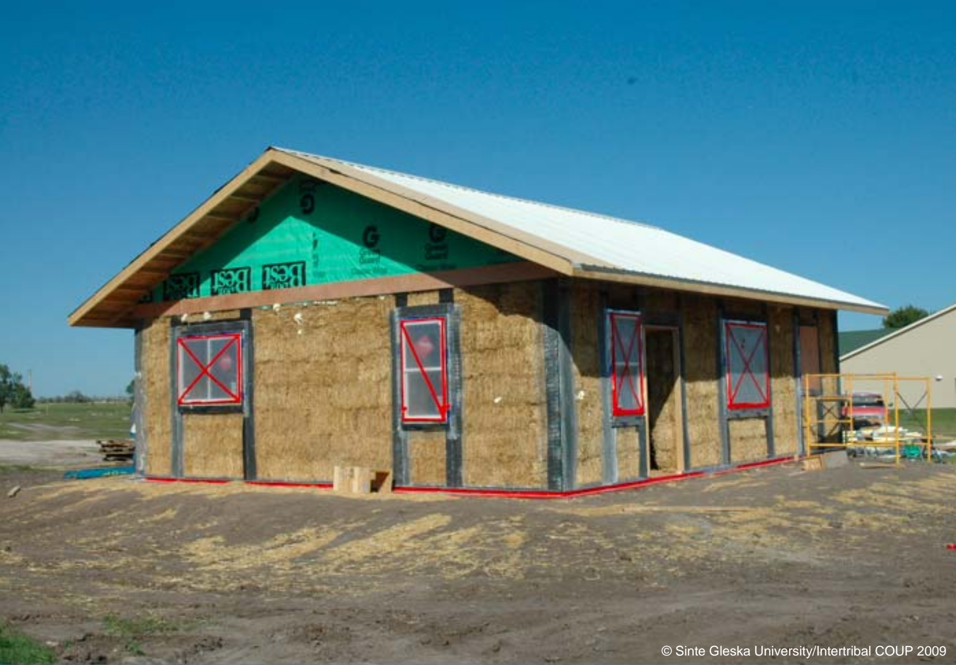
COUP SGU Buffalo Lodge Straw Bale Building prior to Plastering
