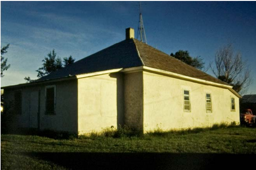
Built in 1921 in southern Todd County, SD
